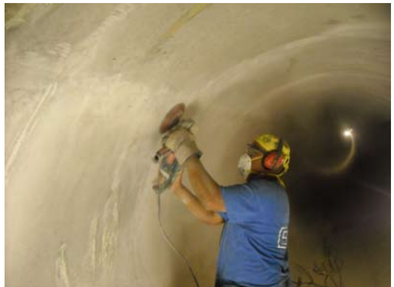
Fig. 4: Prior to installation of the FRP lining, surface preparation included grinding
