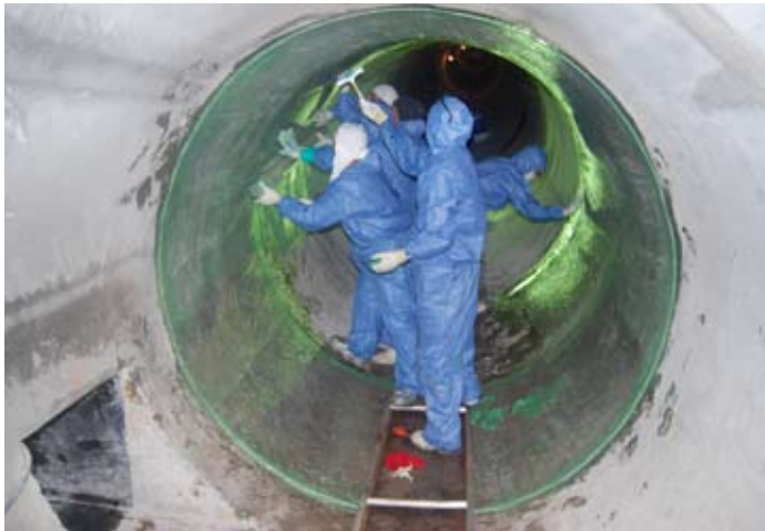
Fig. 5: Installation of FRP sheets on the interior surface of the pipe. An access point is visible at the lower left
