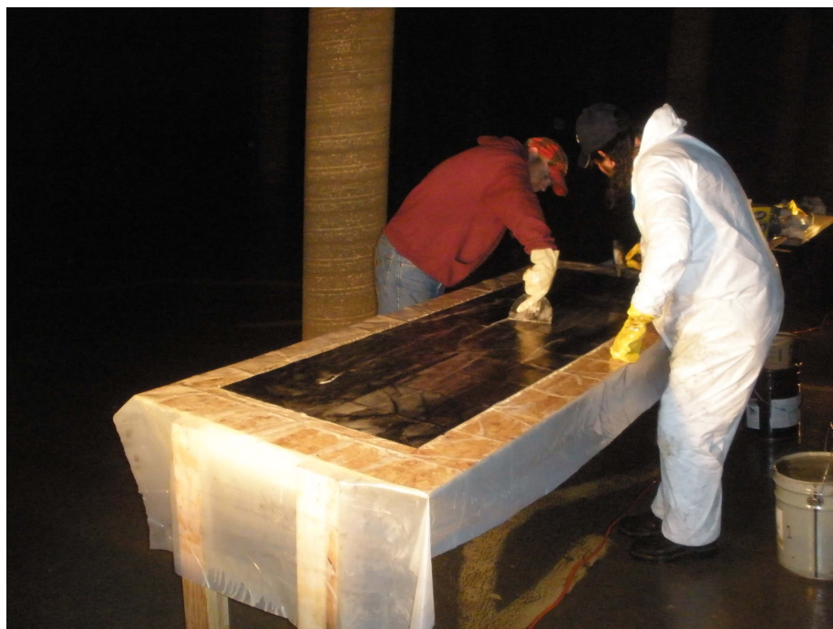
Figure 3: Wetout of carbon fiber textile
