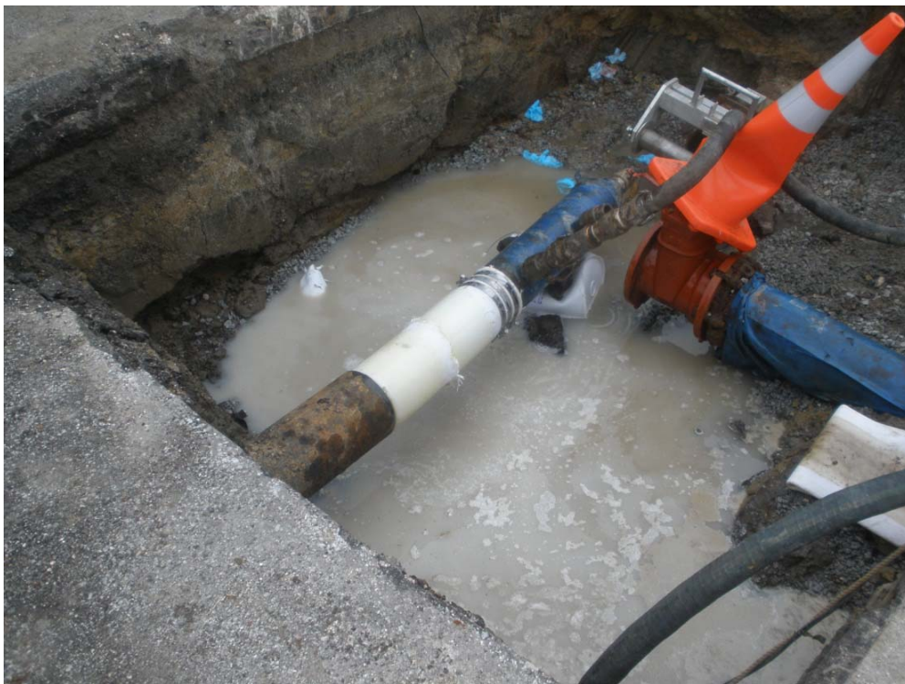
Figure 2: Rounded Aqua-Pipe® after swab pass into receiving "cannon"
