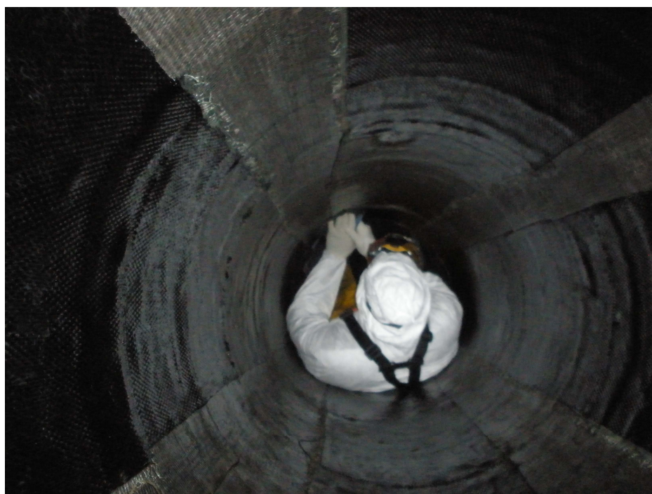
Figure 4: Installation of longitudinal ribs
