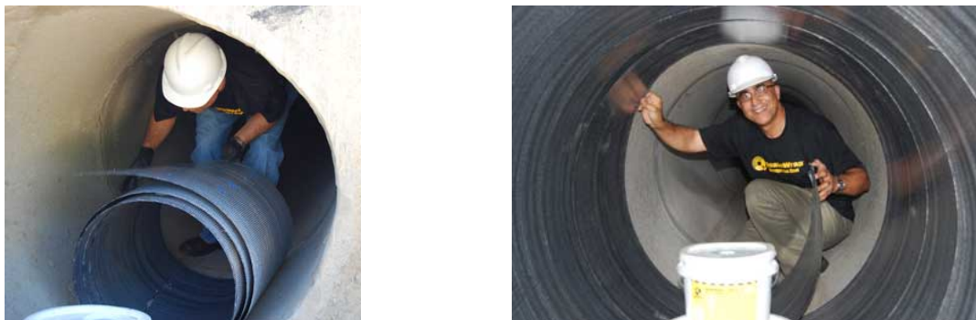
Fig. 5 – PipeMedic™ being taken into the pipe and installed; one size fits all pipe diameters
