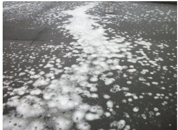
Figure 1. Air bubbles escaping from the pipe
