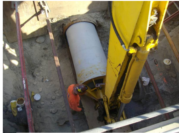
Figure 3. Large Diameter Sliplining
