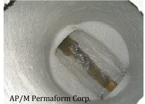
Figure 7. Structural Epoxy Coating
