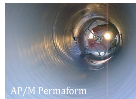
Figure 6. Mortar and Epoxy Composite Lining
