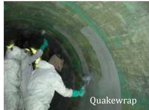
Figure 5. Quakewrap FRP Application
