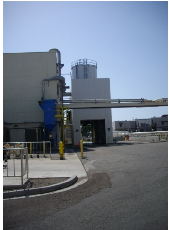
Figure 2. Pellet Loading Station
