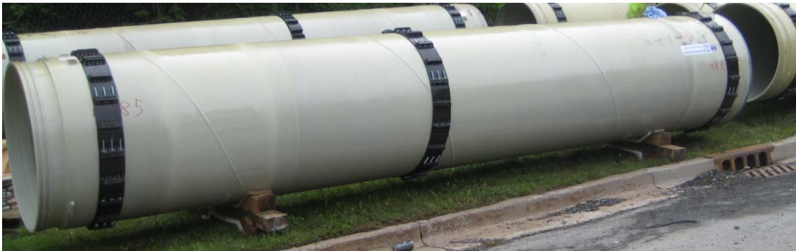
Figure 3: Steel Pipe Liner Sections with Casing Spacers
