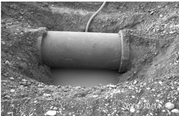
Figure 2 – Concrete Pipe Segment
