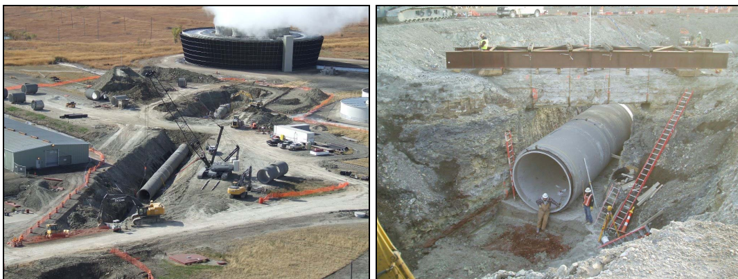
Figure 11 – New Line Installation
