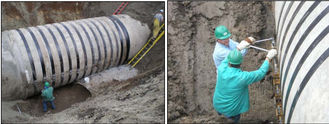
Figure 10 - Steel support band installation
