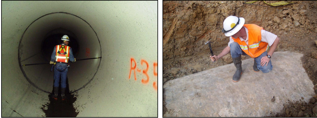
Figure 15 – Internal and External Visual and Sounding
