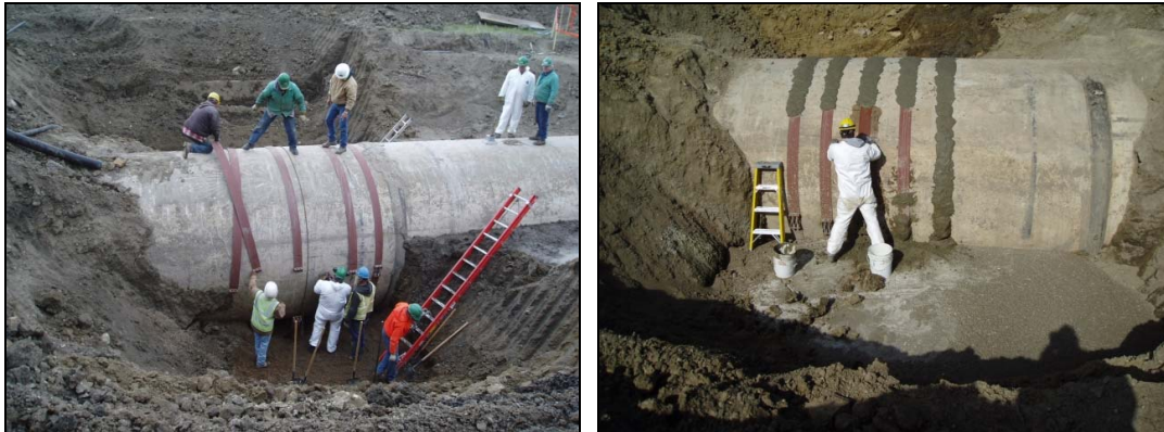
Figure 4- Steel support band installation
