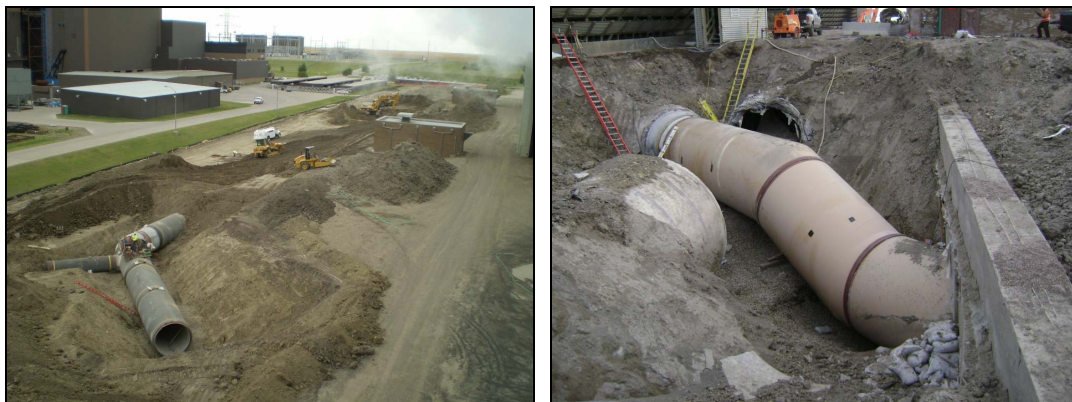
Figure 5 – New Line Installation
