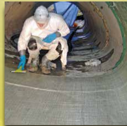
Repair of joints in oval-shaped concrete culvert
