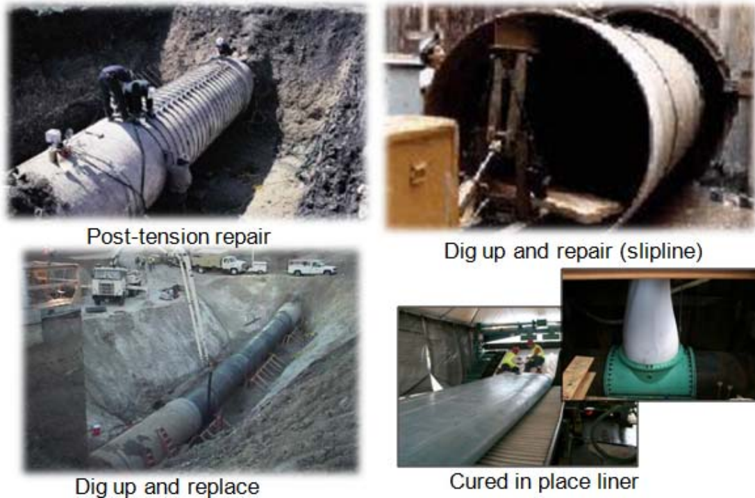
Figure 2. Various solutions for damaged pipelines
