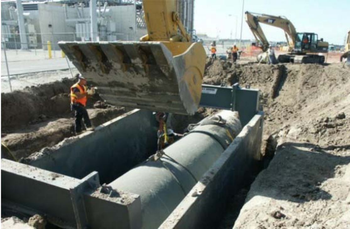
Image 2: Potential Solution – Pipeline Replacement
