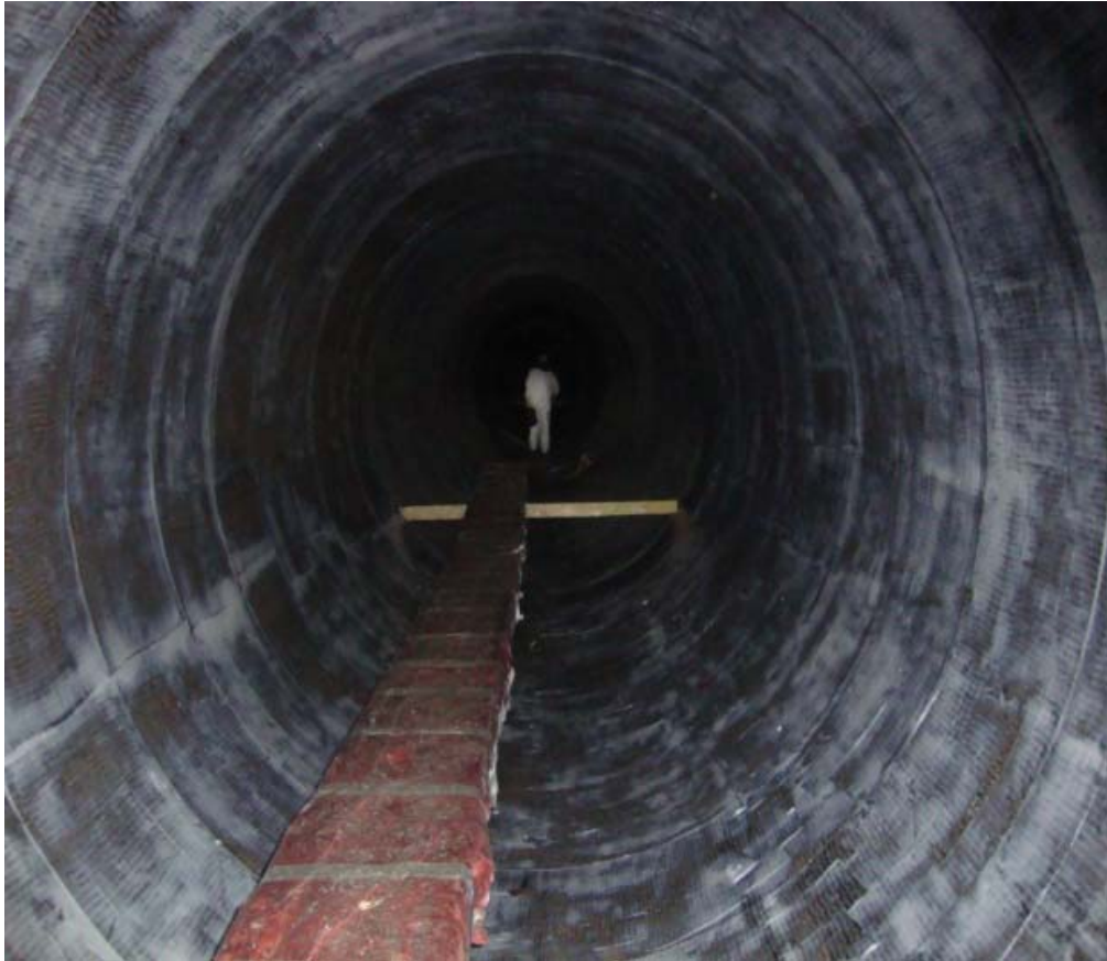
Figure 3. Completed CFRP installation
