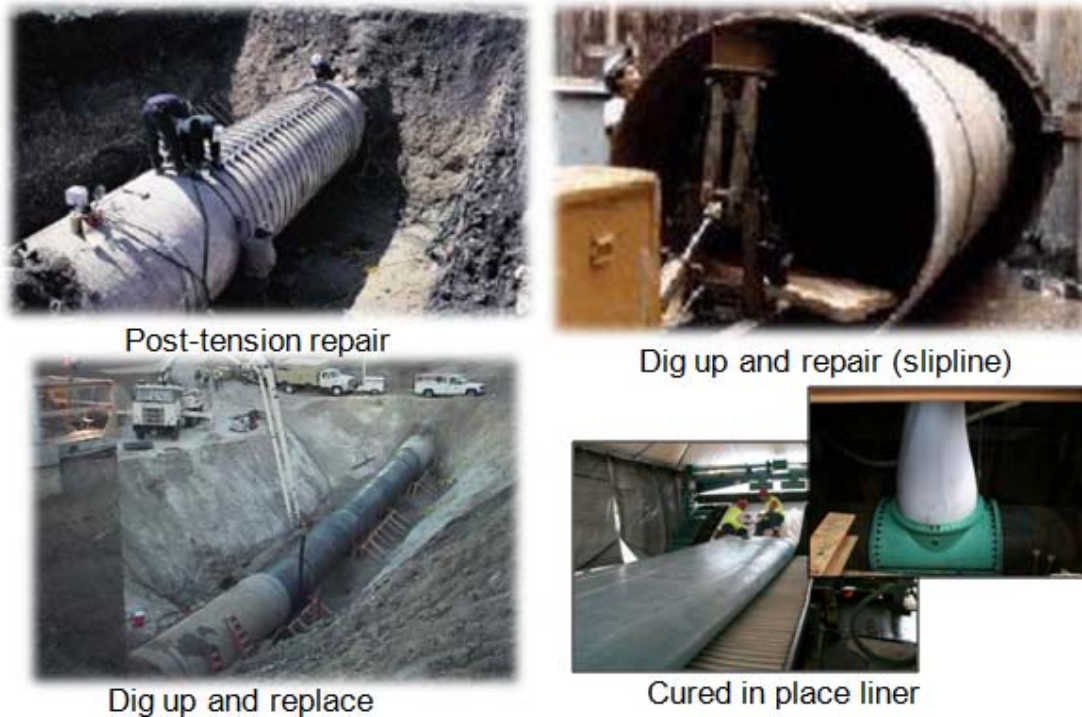
Figure 2. Various solutions for damaged pipelines
