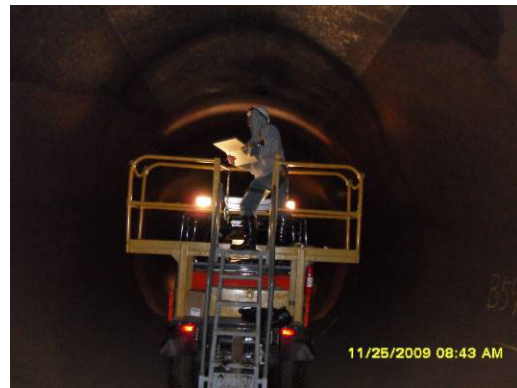
Figure 6 – Inspector on platform
