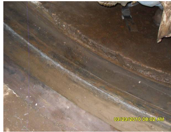
Figure 11 - Observation for Leakage before Mortar Repair
