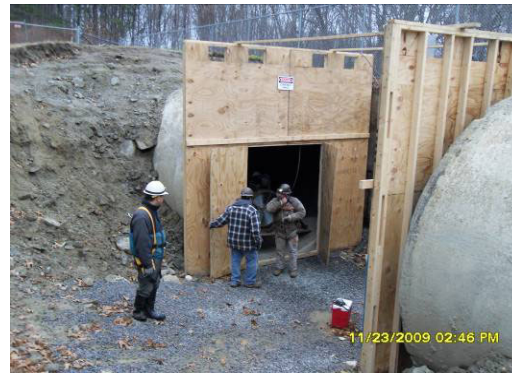
Figure 4 – Access Point (Transition from Segment D and E)
