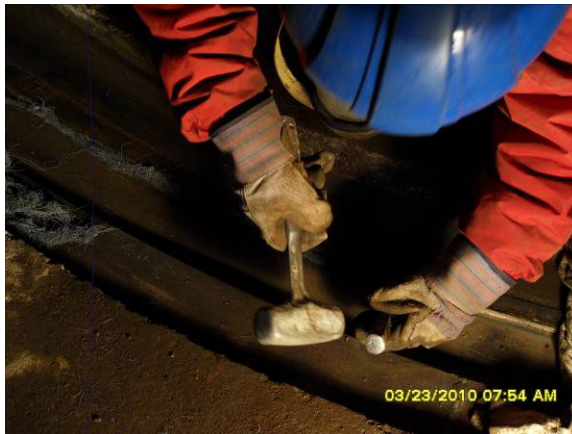
Figure 10 - Lead joint repacking
