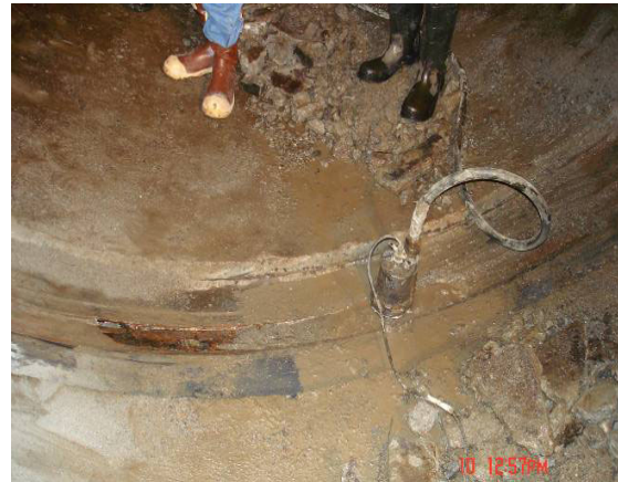
Figure 9 - Mortar Liner Removed
