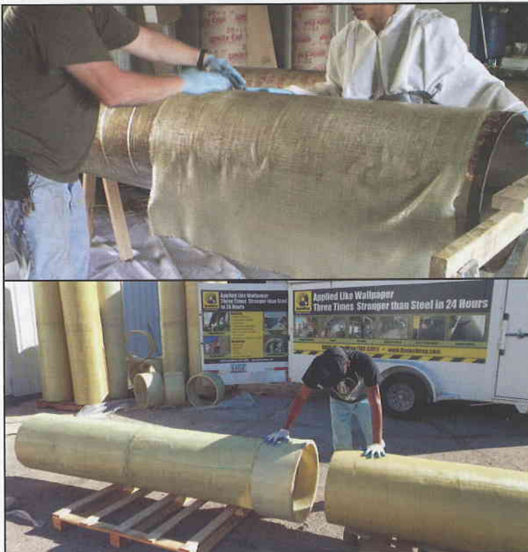
Figure 2. StifPipe is made and connected on site
