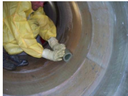
Figure 1. Repair of pipes with wet layup FRP
