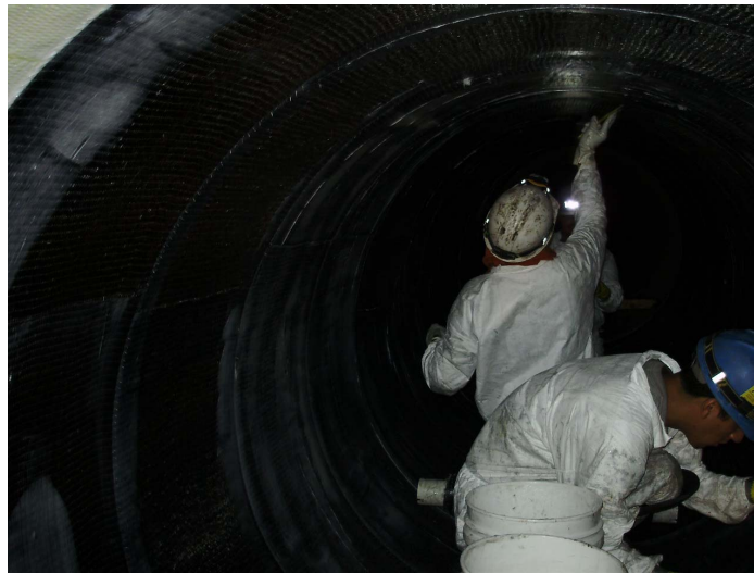
Figure 2. Interior of Denver Water Steel Pipe
