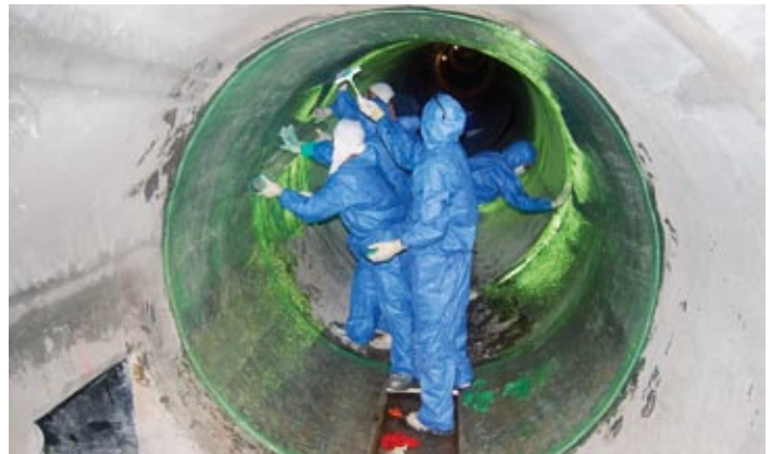
Fig. 6: Installation of FRP sheets on the interior surface of the pipeline
