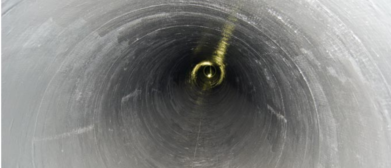
Fig. 8: Completed segment of pipeline prior to testing
