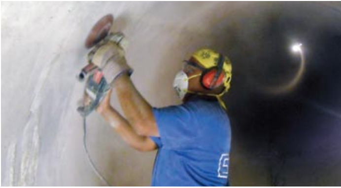
Fig. 4: Preparation work prior to installation of FRP lining
