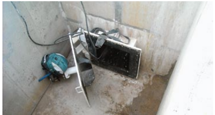
Fig. 5: Typical 2 ft. x 2 ft. access point
