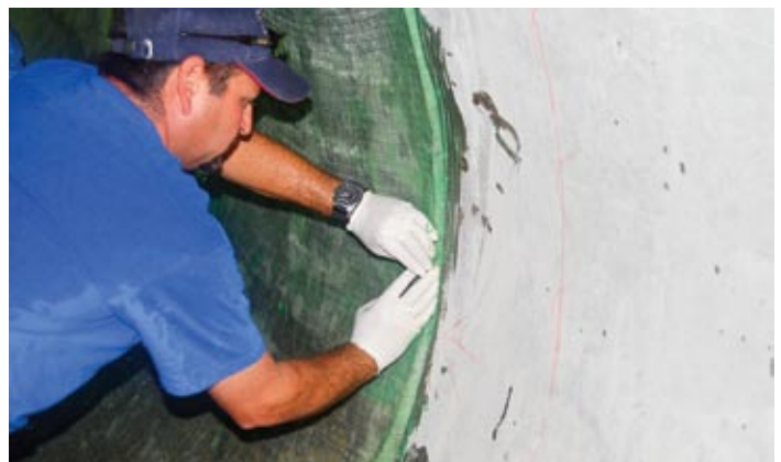
Fig. 7: Construction joint of FRP lining
