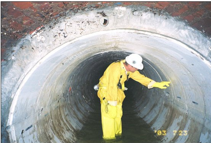
Figure 10: Inspecting the 40 ft section
