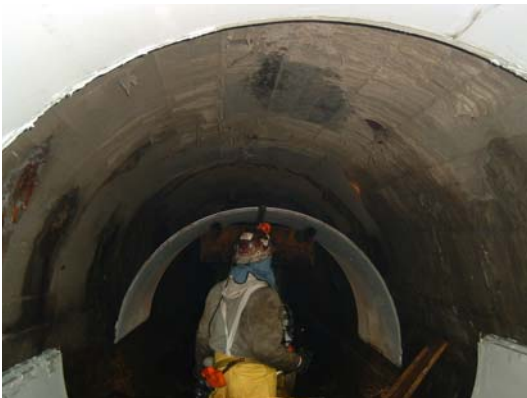
Figure 7: Transporting a panel in 9 ft. sewer
