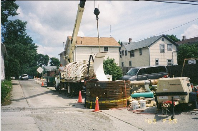
Figure 9: Lowering a panel into shaft
