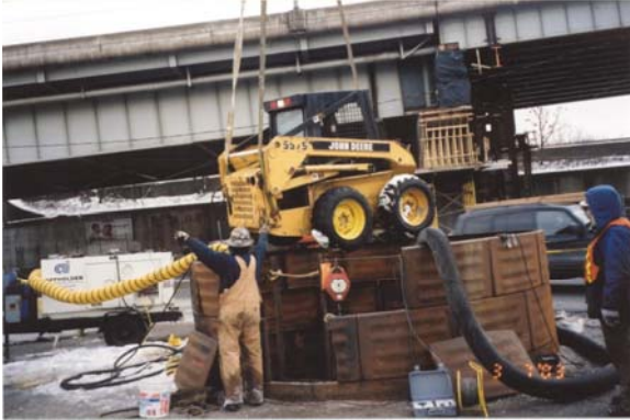
Figure 6: Lowering equipment into shaft
