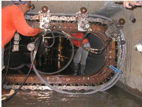
Figure 4. Winding the Liner in the Emergency Bypass Channel
