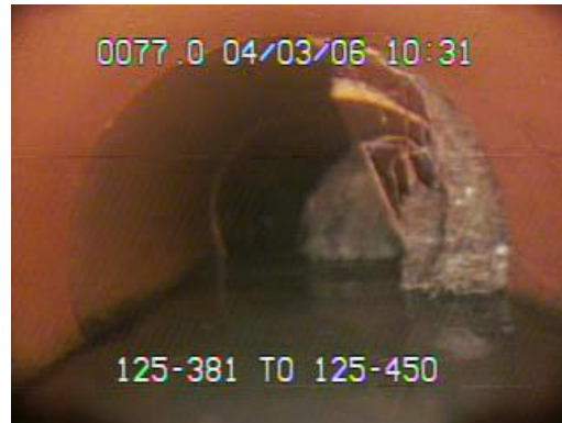
Figure 9. Example of roots in a broken pipe.
