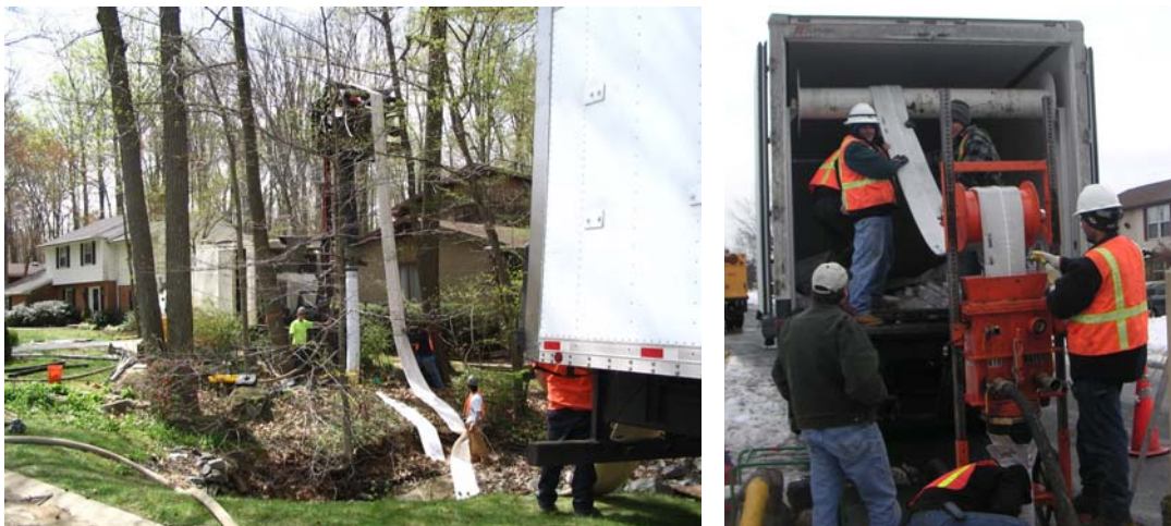
Figure 3. Inversion liner (left: difficult water inversion setup; right: typical roadway air inversion setup).
