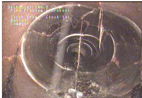
Figure 5. Example of pipe with a greater than 10% ovality.
