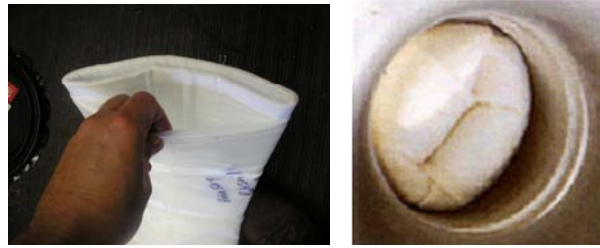
Figure 2. Inversion liner (left: flexible tube with coating on “exterior” (prior to inversion) of the liner; right: liner as it is be inverted in the pipe).
