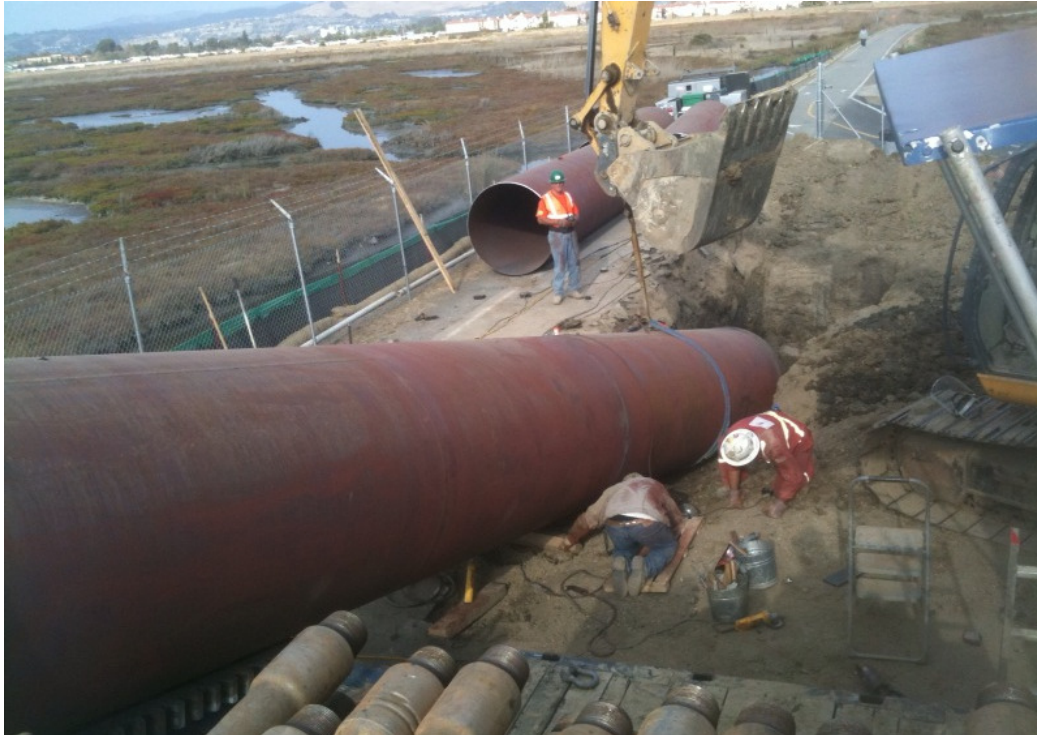
Figure 5. Conductor Casing Being Installed at Entry Point
