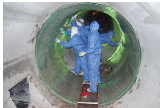
Figure 5: Installation of FRP sheets on the interior surface of the pipeline.
