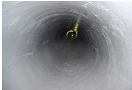
Figure 6: Completed segment of pipeline prior to testing.
