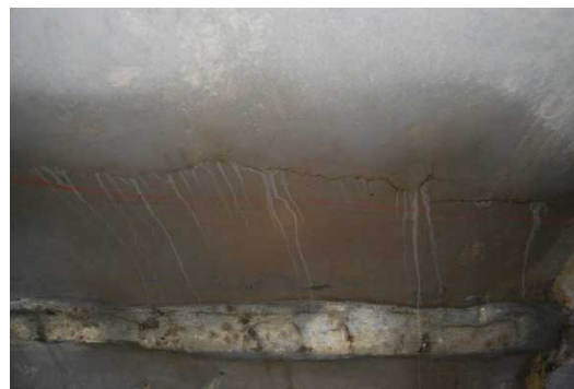
Figure 3: Water seeping into pipeline
