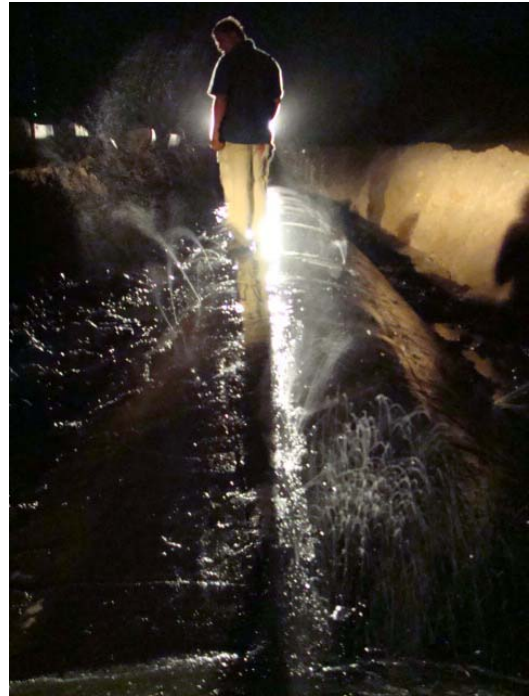
Figure 2: Leaking after conventional crack sealing
