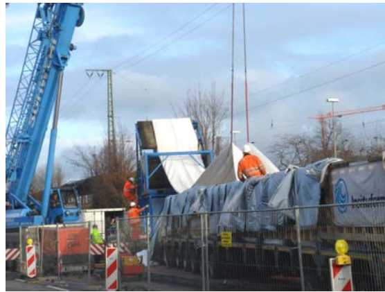
Figure 22. Installation of the CIPP lining
