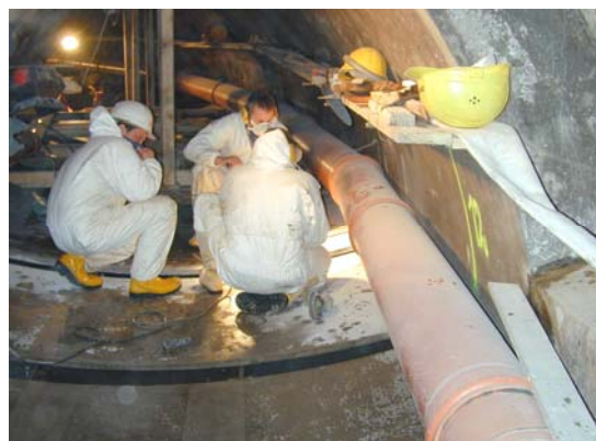
Figure 20. Assembly of the liner elements, bonding
