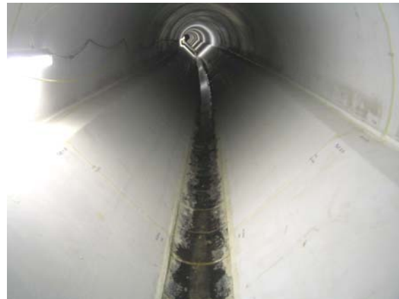
Figure 16. Sewer in Düsseldorf, Germany after renovation (Photos: H.I. Hammer)
