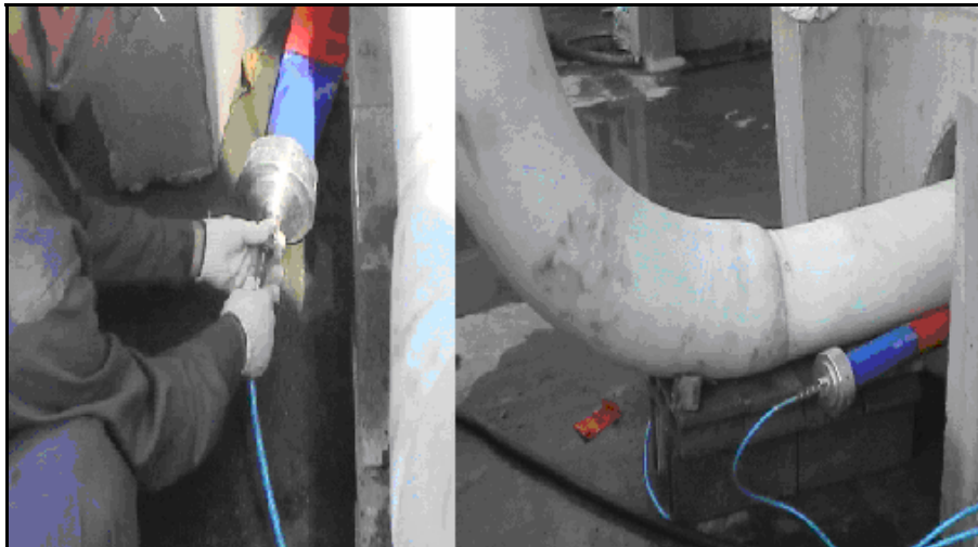
Figure 6. Air Pressure Inflating Tube after Inversion Process
