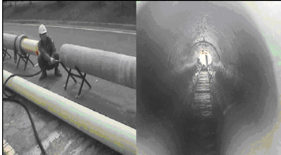
Figure 7. Mortar Injection and Completed shape of MSCIPP
