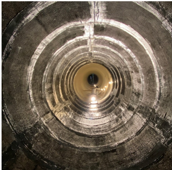
Complete CFRP liner prior to applying top coat.
