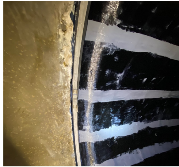
Compression seal (Weko) at the end termination.
