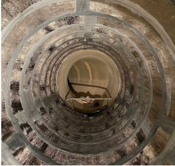
CFRP layers being applied with extra tack coat along the seams.
