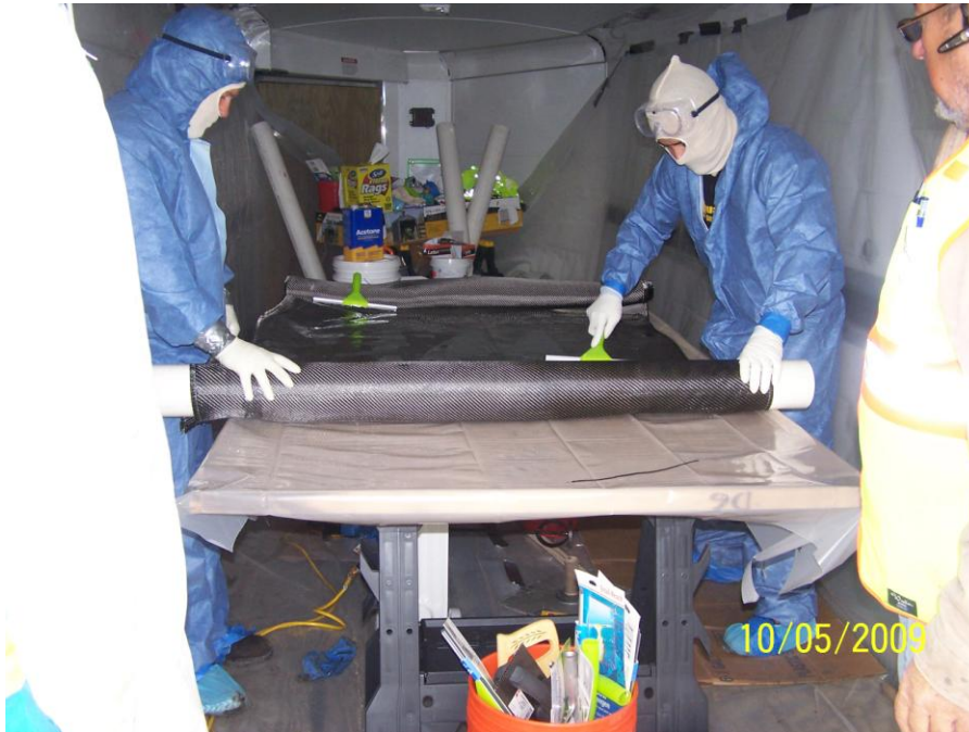
Photo 142: QuakeWrap being saturated before installation
