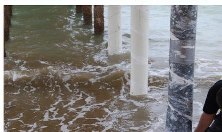
**Figure 6: Construction of a continuous PipeMedic™ jacket around an existing steel pipe with super laminate; filling the annular space with grout, and view of retrofitted piles.**
