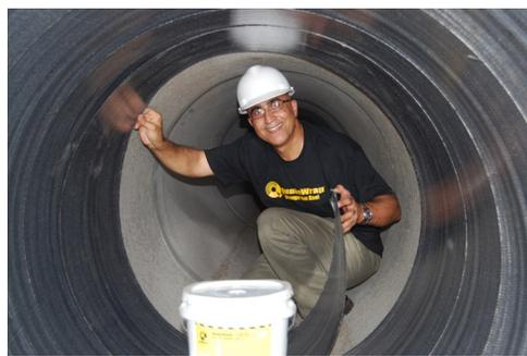
**Figure 3:** Coiled PipeMedic™ laminate being taken into a pipe and bonded to the pipe surface.
