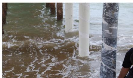
**Figure 6: Construction of a continuous PipeMedic™ jacket around an existing steel pipe with super laminate; filling the annular space with grout, and view of retrofitted piles.**
