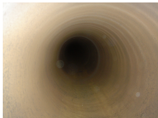
Figure 18. Pipeline ID fully cleaned.
