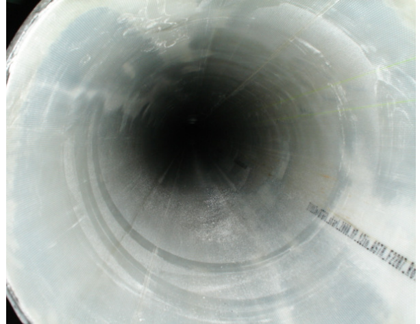
Figure 22. Completed liner installation with the FRP laminate through the drip pot.
