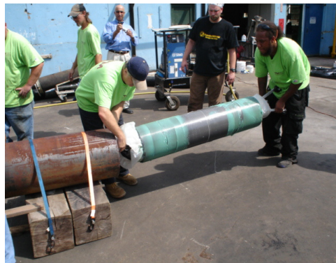
Figure 6. Insertion into pipe section.
