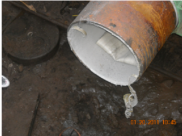
Figure 21. Excess liner being trimmed at pipe-ends.
