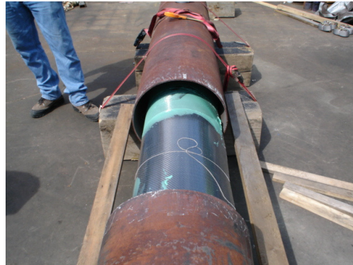
Figure 7. Laminate in position and pig being inflated.
