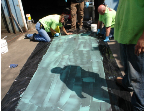
Figure 4. Adhesive application.
