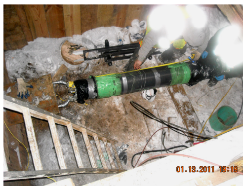
Figure 19. Inflatable pig/laminate being inserted.
