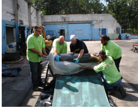
Figure 5. Laminate installed onto inflatable pig.
