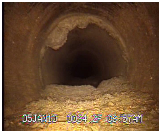
Figure 15. Heavily debris-laden pipe ID.
