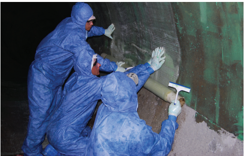
Figure 7(c) Transitions between top and bottom half installation
