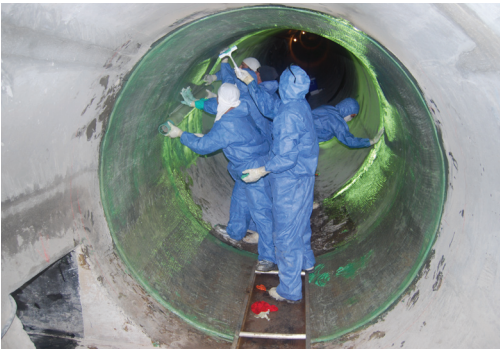
Figure 7(b): Installation of FRP lining
