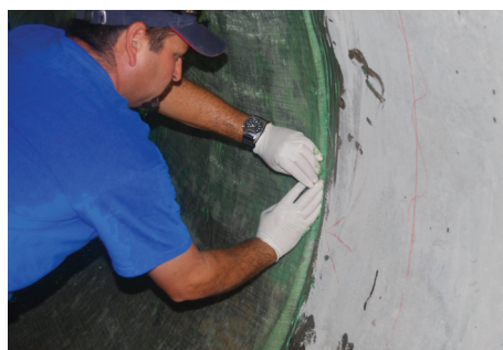
Figure 8: Construction joint of FRP lining
