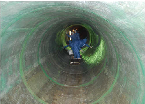
Figure 7(d): Detailing of FRP lining
