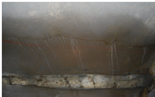
Figure 3: Seepage water draining into pipeline
