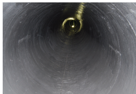
Figure 10: Completed segment of the FRP installation
