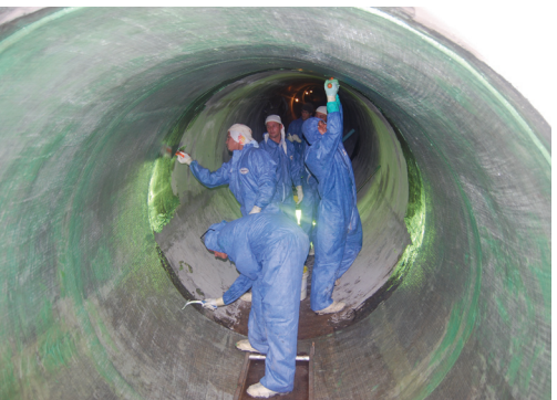
Figure 7(a): Epoxy paste installation on top half of pipeline
