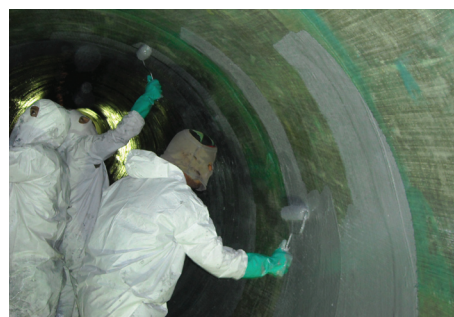
Figure 9: Application of epoxy top coat
