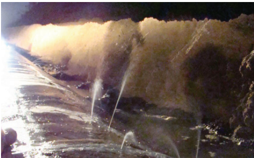
Figure 2: Leaking after conventional crack sealing
