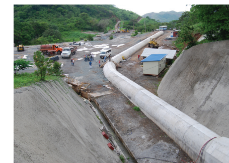
Figure 1: Above ground segment of the "El Encanto" pipeline
