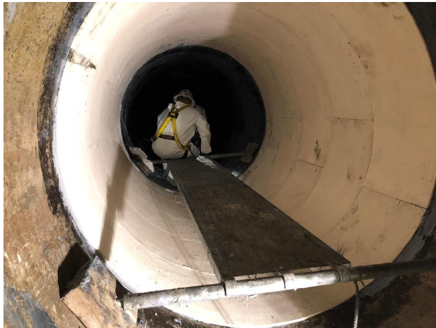
Figure 3. Installation of .57 in. thick StifPipe® inside the 66-inch RCP.
