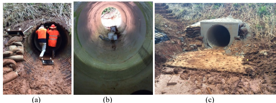
Fig. 4. (a) Caster trolleys inside the culvert allowed pushing lightweight StifPipe® segments by hand into the culvert; (b) joining of segments with wet layup; (c) finished project.
