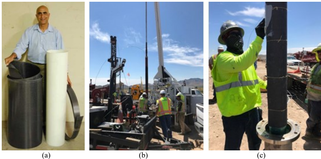
Fig. 6. Application of SuperLaminate to repair of pressure pipes: (a) Samples of SuperLaminate, (b) Site location for 500m (1600 ft) long pipe, and (c) SuperLaminate wrapped around a packer to be sent into the well.
