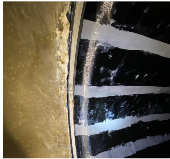
Compression seal (Weko) at the end termination.
