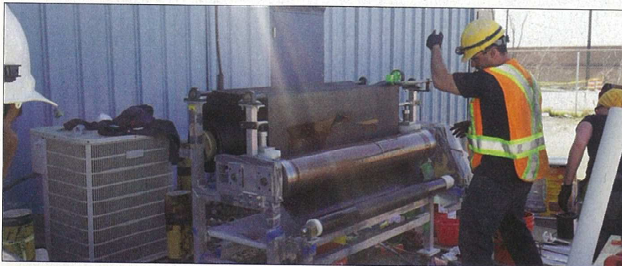
↑ Figure 1. Carbon fabric being saturated with epoxy resin through a saturating machine.
