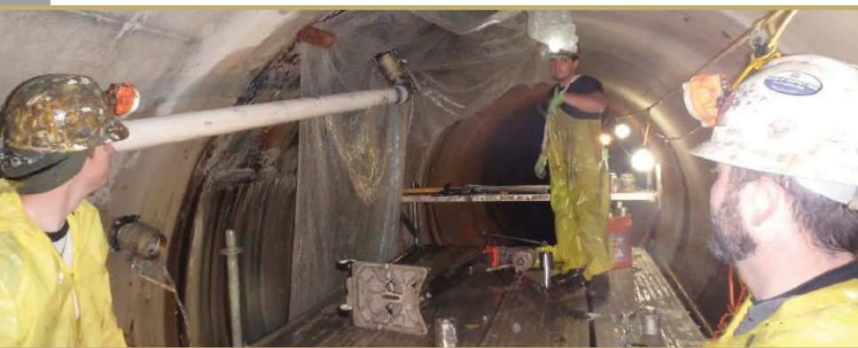
Figure 1. Groundwater relief port installation by the General Contractor, PCi Roads.
