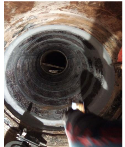
Interior of the pipe after CFRP lining
