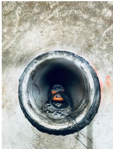
Interior of the pipe before CFRP lining
